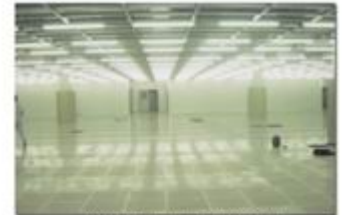
1000 级净化车间防静电地板与通风系统安装图 Installation of the coating aluminum solid panel and grating panel in 1000 class cleanroom
